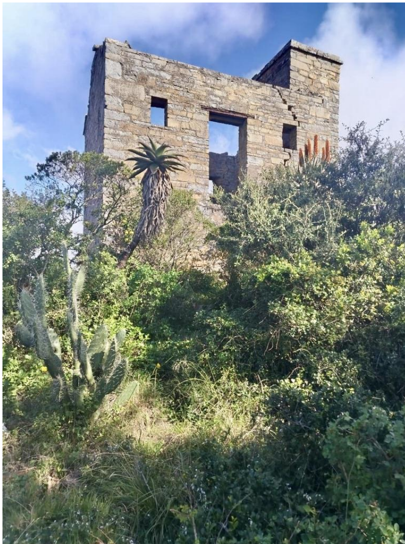
Left: remains of the tower at Governor's Kop, 2024
